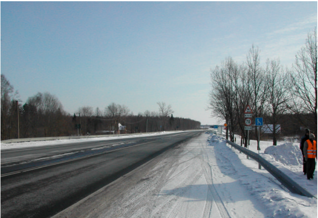
T-2 towards Tartu. Visibility is limited by trees, signs and shelter
